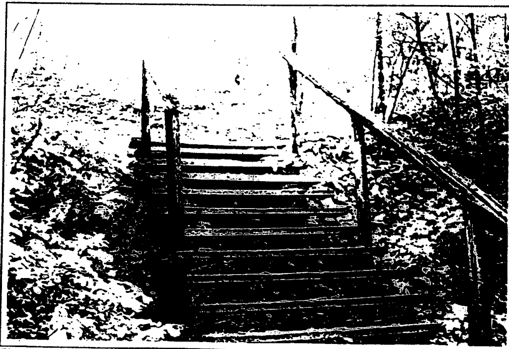
Figure 33: Wooden staircase providing access to the Lake Residence Access Road.
