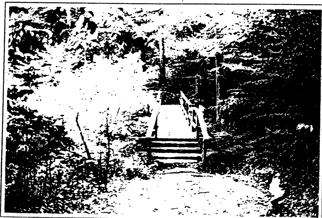
Figure 15: Wooden bridge over the Mill River north of the Cascades, looking west.
